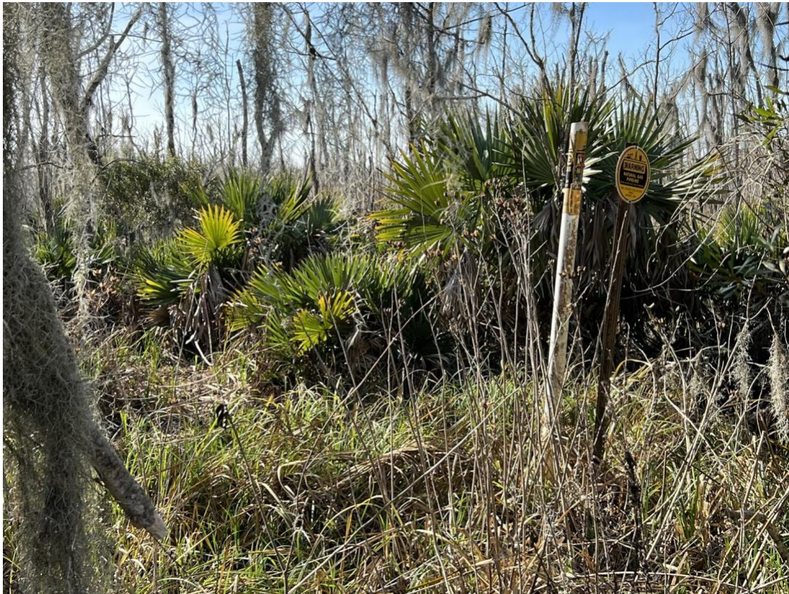
Natural gas pipeline infrastructure running through the Mandalay National Wildlife Refuge in Houma, LA. Photo by author, February 2024.
